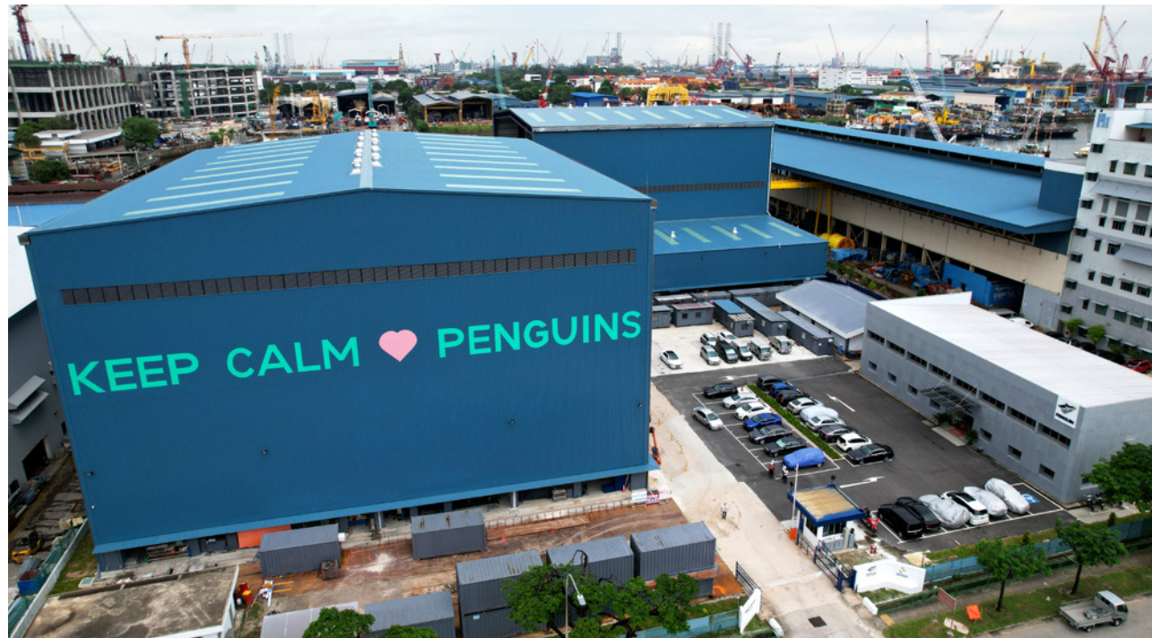
Penguin's newly developed shipbuilding and repair hub at 21 Tuas Road in Singapore.
