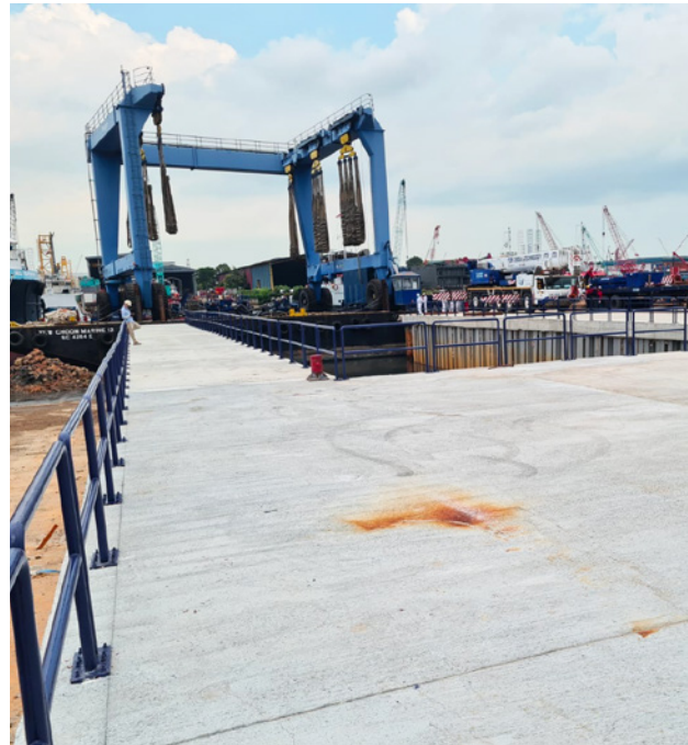
Newly built 50m piers for our marine travel lift in Singapore
