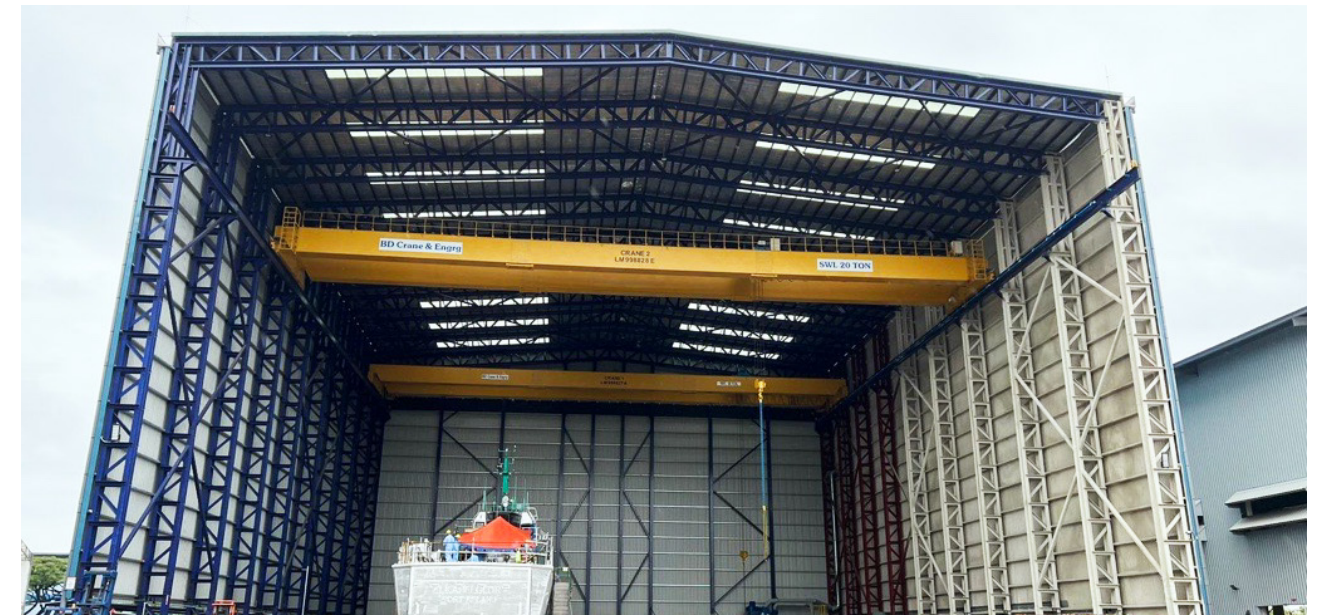
One of two new workshops at 21 Tuas Road
