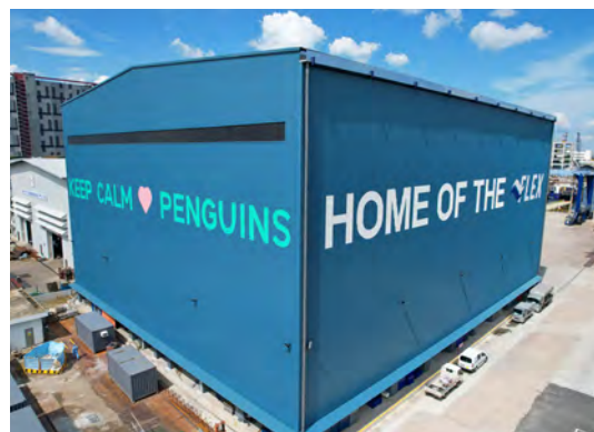
Penguin's headquarters at 21 Tuas Road in Singapore.
