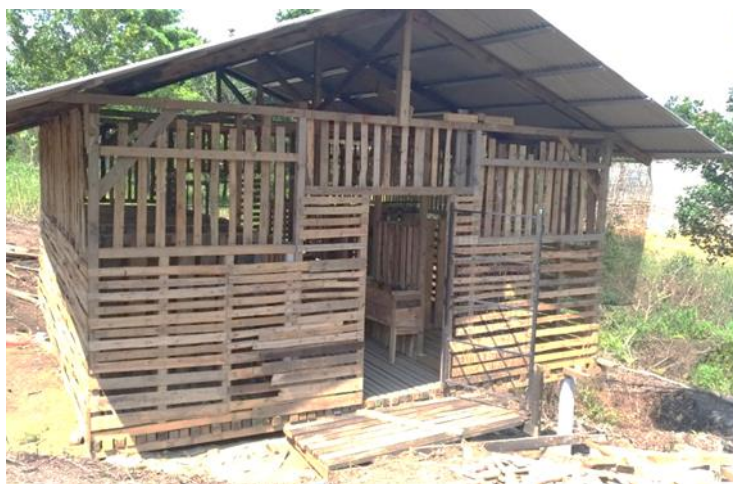
Goat pens constructed from recycled timber in Batam
